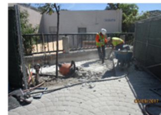
LBTC Bridge Repair Project
